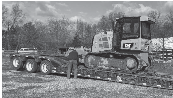
Construction Equipment Arriving on Site
